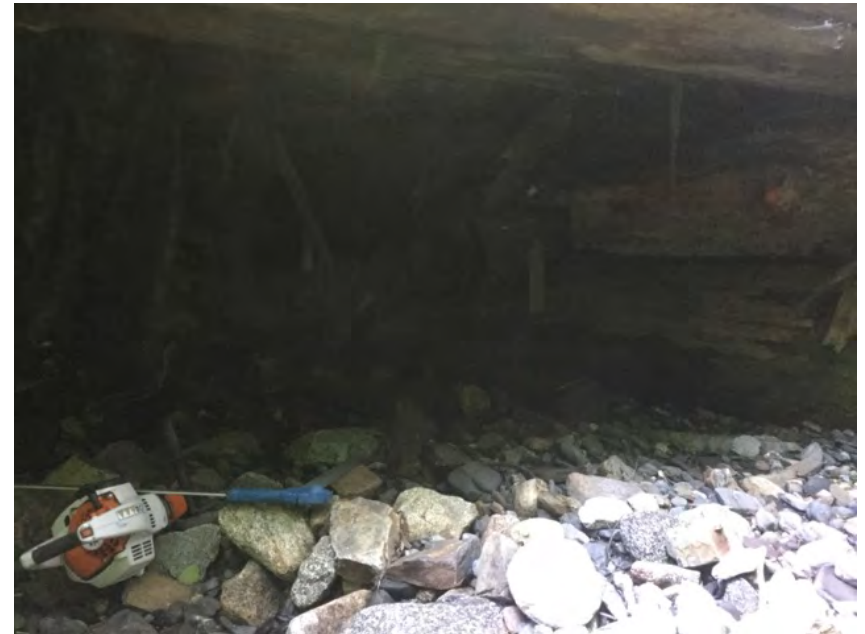
Right Bank Abutment when facing downstream
