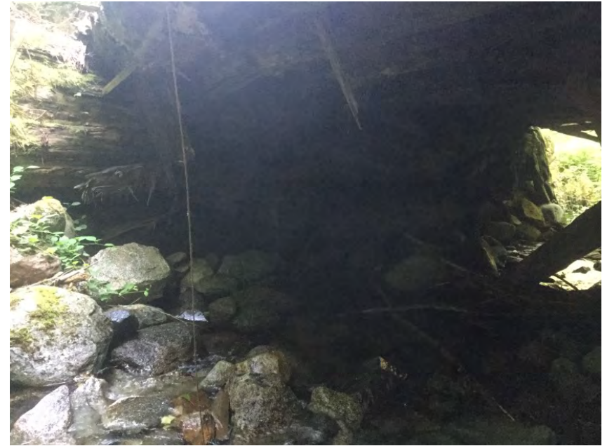
Left Bank Abutment when facing downstream
